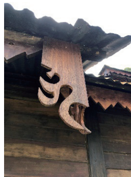
Figure 16. Lizard's Tail Roof Fascia Board
