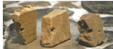
Picture 8. Holes on Preah Ko Brick (source : The Pre-Angkorian Temple of Preah Ko)
