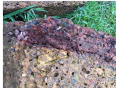
Picture 29. Deteriorated Condition by Iron Oxide
