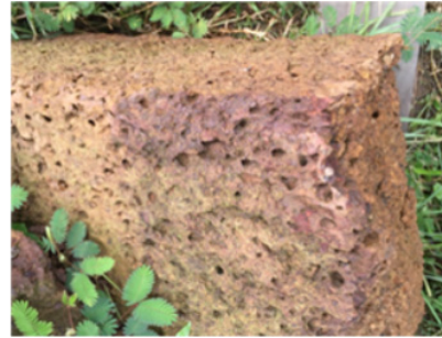
Picture 29. Deteriorated Condition by Iron Oxide
